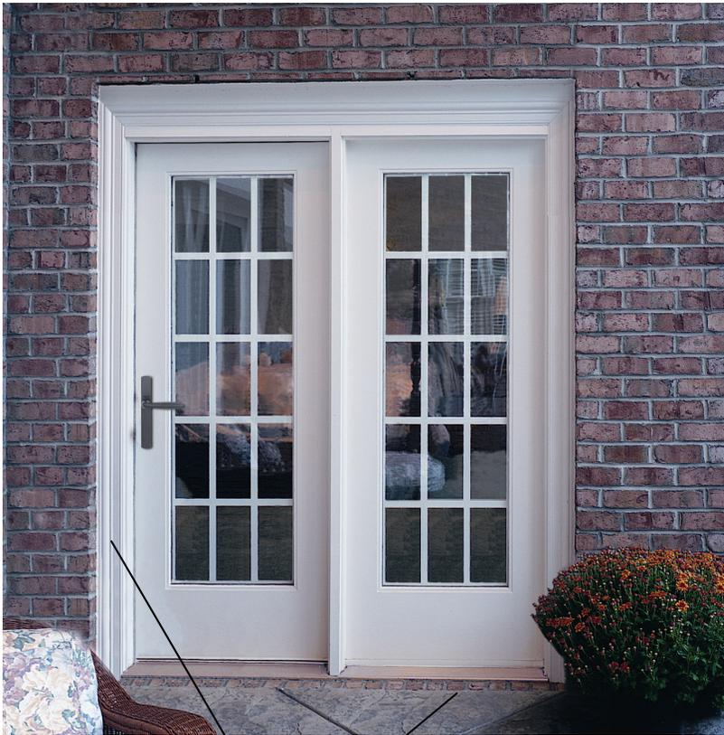
Figure #5 Must caulk around the entire perimeter of the door
