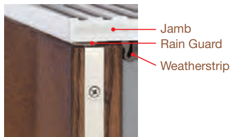
Top of door; exterior view.
